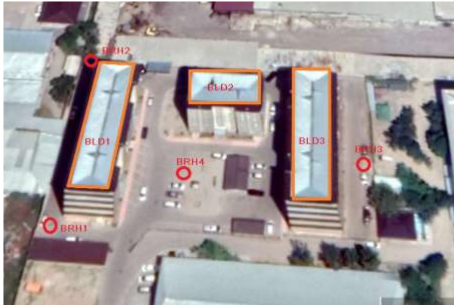
Fig. 1.4.2. Monitoring test site consisting of wells (red circles) and buildings (orange rectangles)
